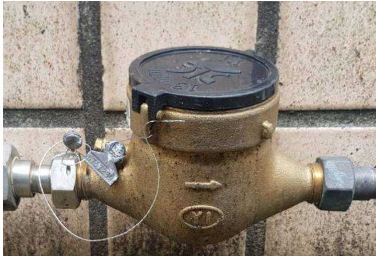
Traditional Water Meter
